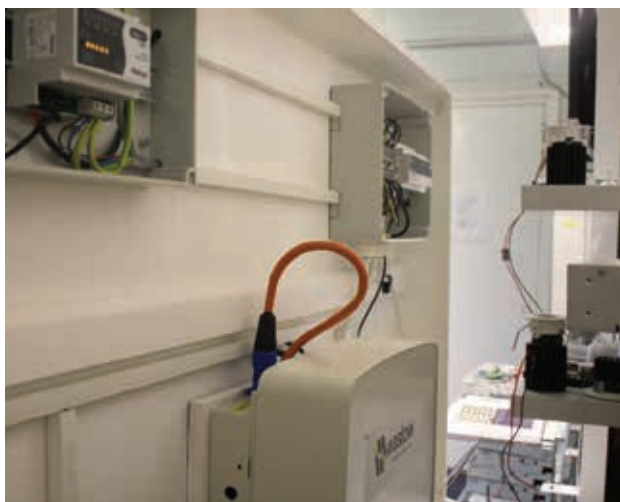
The Hoare Lea/Moxia Energy demonstration project – battery and DC voltage converter enclosures
